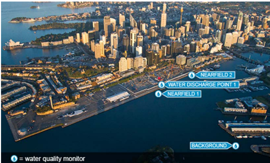
Approximate locations of water monitoring equipment
