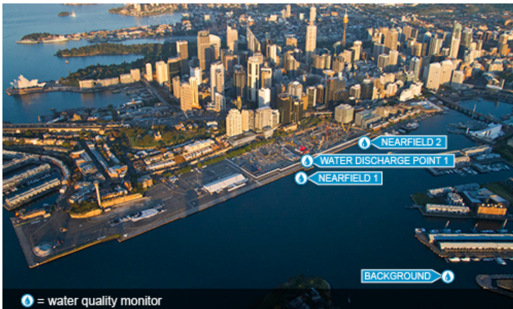
Approximate locations of water monitoring equipment
